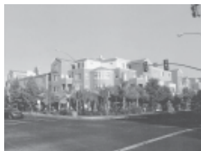
City Center Plaza, Redwood City
